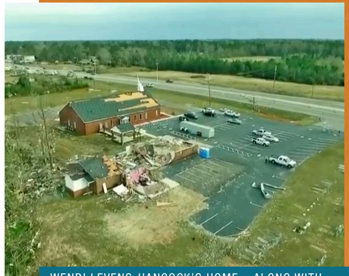
WENDI LEVENS-HANCOCK'S HOME – ALONG WITH MANY NEARBY STRUCTURES – WAS DAMAGED WHEN A TORNADO HIT HATTIESBURG, MISS.
